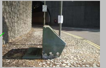
CUILFAIL TUNNEL NORTH
